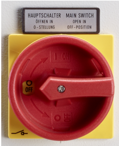
Fig. 2: Electrical main switch
